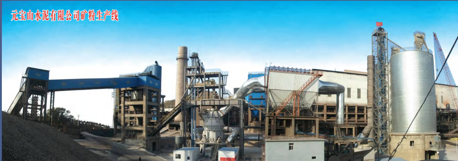
矿渣立磨生产线 slag grinding vertical mill production line
