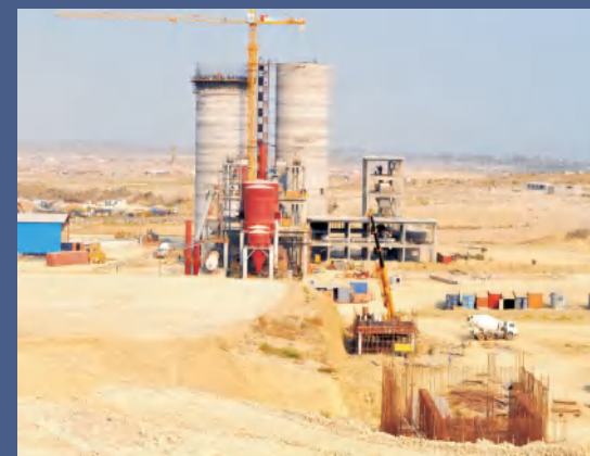
安哥拉水泥厂施工现场 Construction site of Angola Cement Plant
