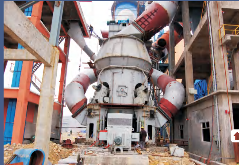
水泥原料立磨安装现场 Cement raw material vertical mill installation site
